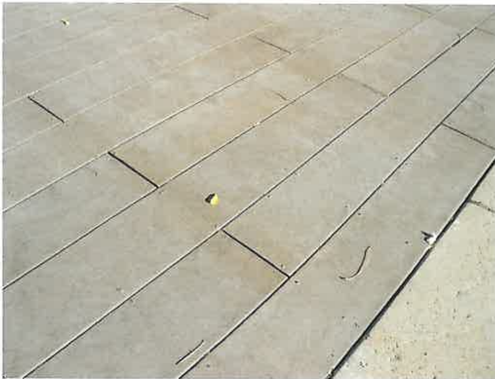
BLACK DIAMOND PLAZA TRAIL – Bridge Surface Replacement Project
