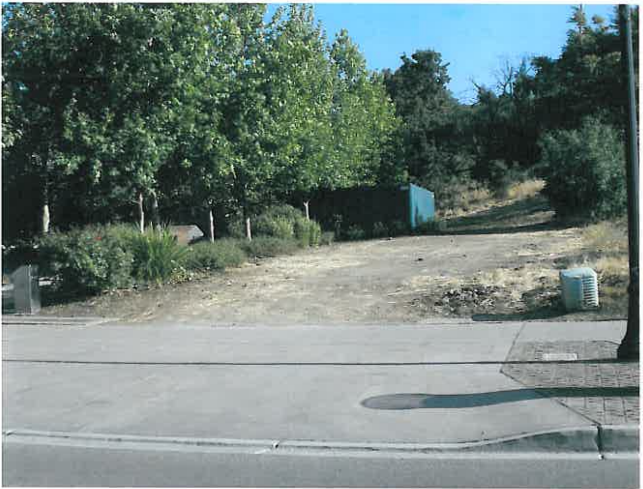
DOWNTOWN WELL WATER HOLDING TANK/ENCLOSURE
